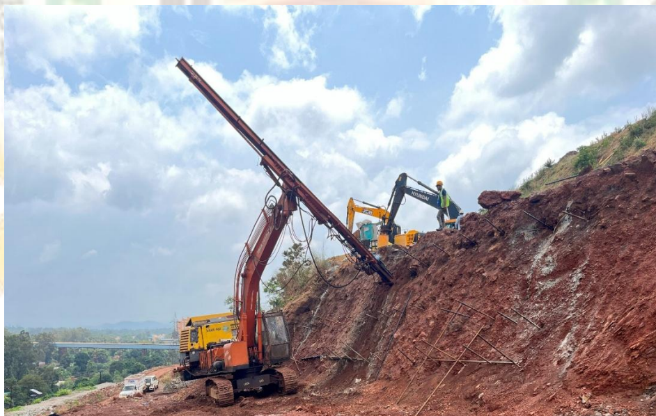
Fig. 4: Rock nailing work at slope site
