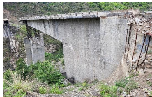
Fig.8: Wangchu Bridge, 204 m span PSC Cantilever Bridge, Project Dantak, 19 Border Roads Task Force (BRTF), Bhutan which had collapsed on 9 th February, 2021 where nine people died
