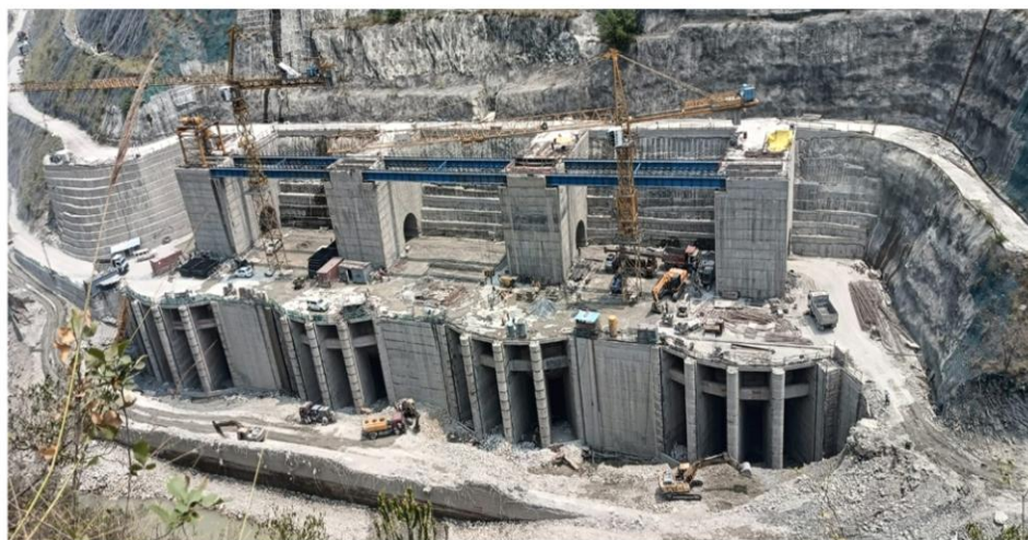
Site photograph of TRT Outfall Structures of Pump Storage Power Plant Project, Tehri showing completion of critical rock excavation and associated rock mass support
