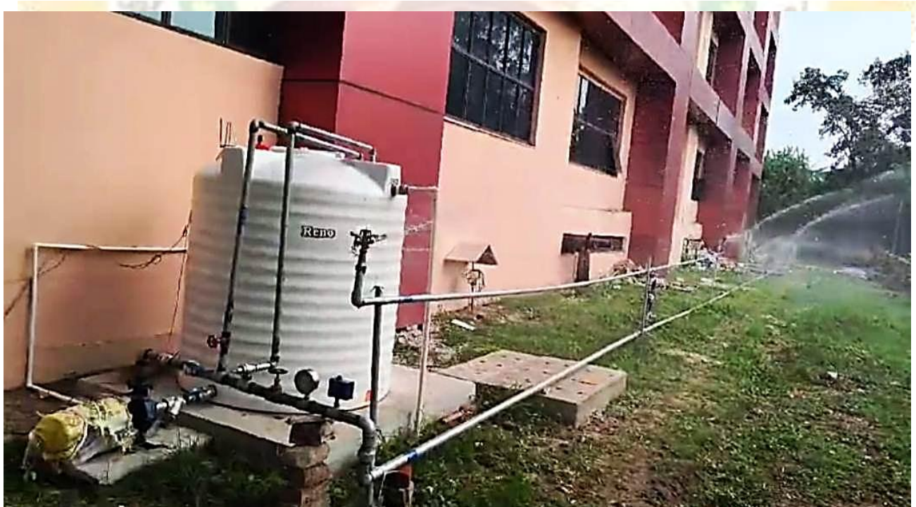
Fig. 1: View of the installed automatic wireless sprinkling system
