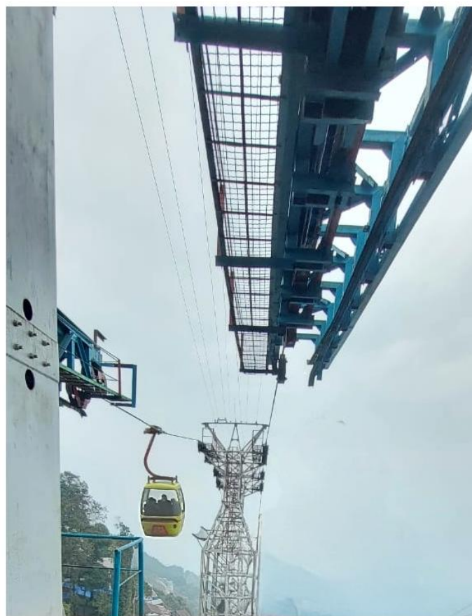
Evaluation of 4.6 KM long haulage rope carried out at DRV Ropeway installation at Darjeeling, West Bengal.
